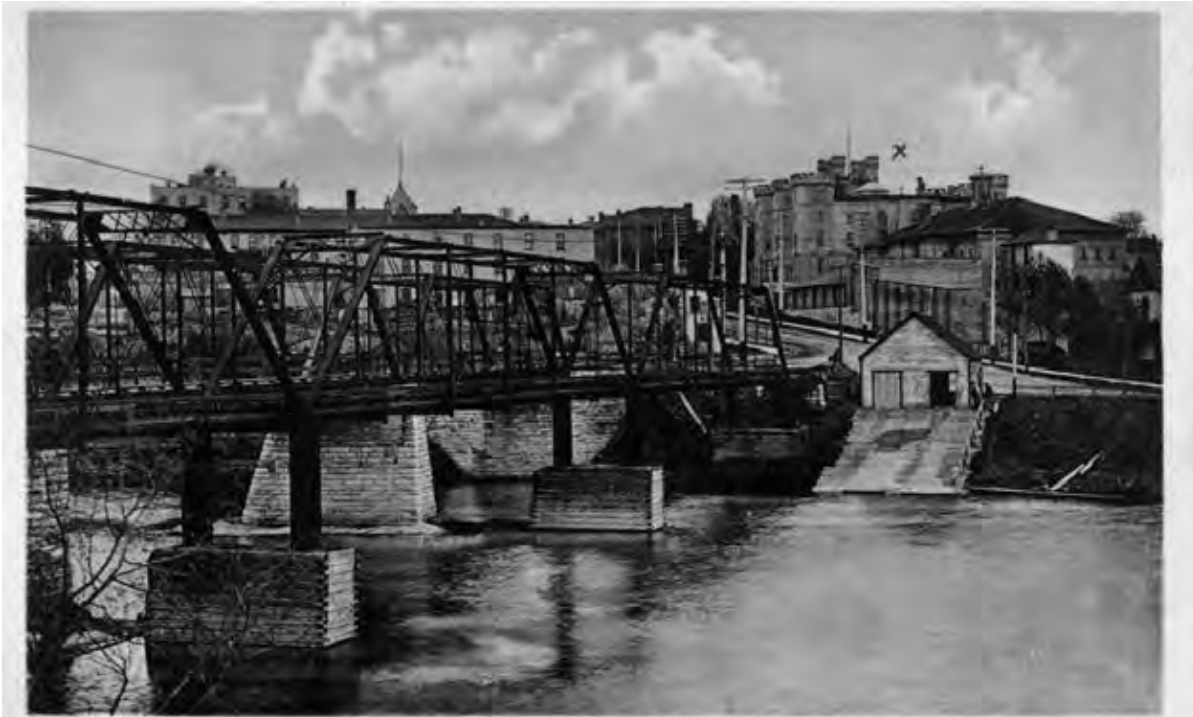
Kensington Bridge showing Jail, London, Ont.
