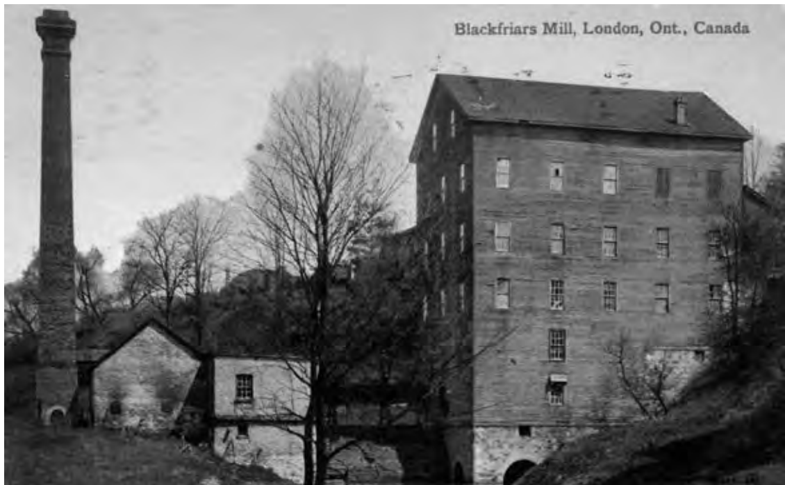
Blackfriar's Mill, London, Ont., Canada.
