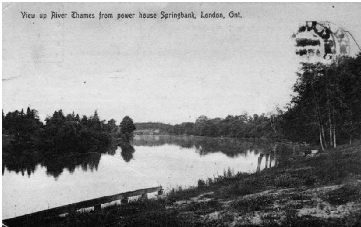
View up River Thames from power house, Springbank. Publisher: Red Star News
