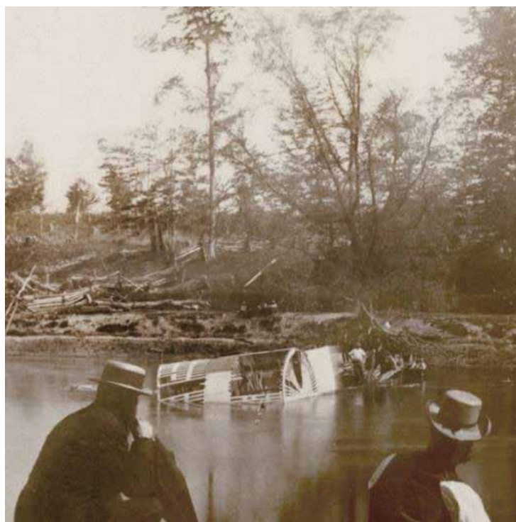
Viewing the Wreck from the London Township Side of the River the Next Day
