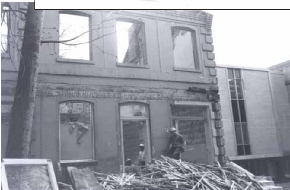
Demolition of 325 Queens Avenue, 1967
