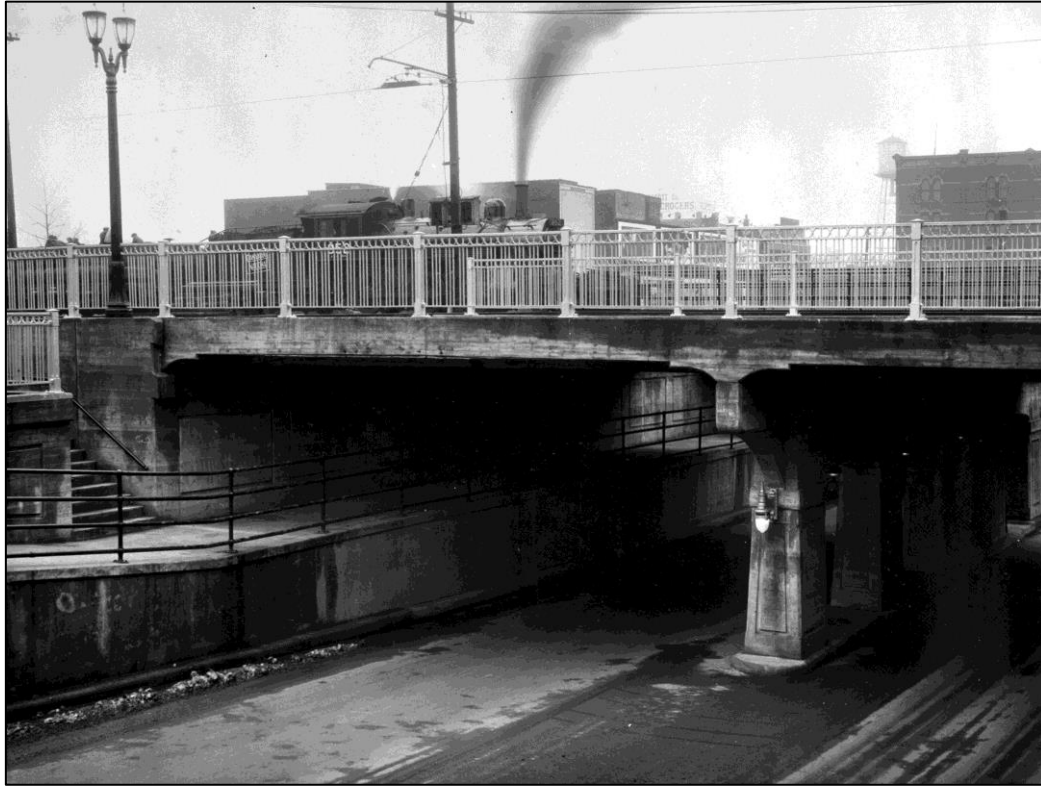
Richmond Street exit to Bathurst Street looking north, Dec 1931. On the bridge is train 852 2-6-0 E7a. Courtesy of The Canadian Museum of Science and Technology (STR29576).
