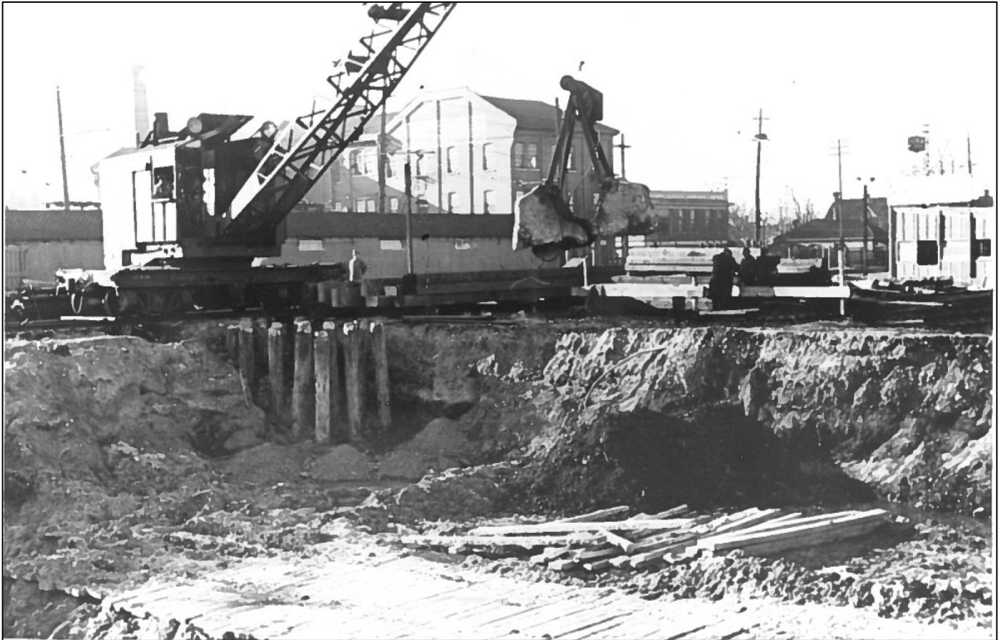
Construction begins at Wellington and Richmond Streets 1931. Courtesy of Western Archives, Western University (RC41958).
