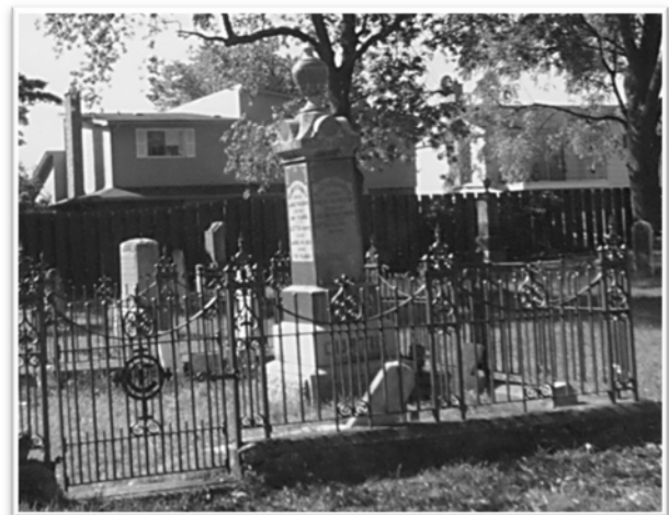
Curtis monument Aug. 17, 2009. Notice the tilt on this large stone inside the fenced enclosure.
