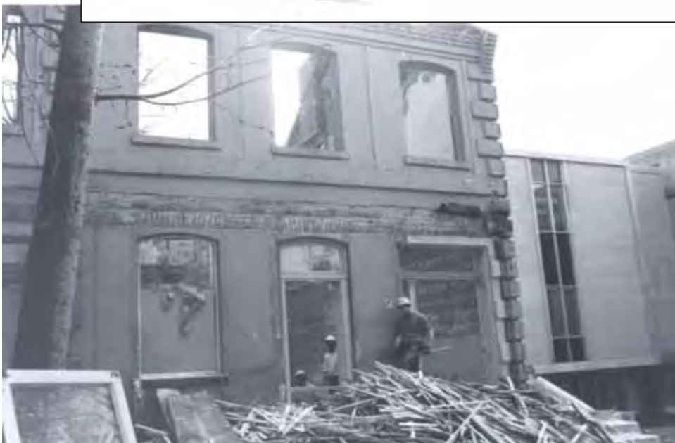
Demolition of 325 Queens Avenue, 1967
