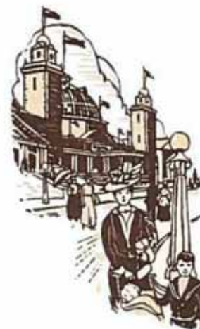
Dominion Government Building, Constructed in 1912
